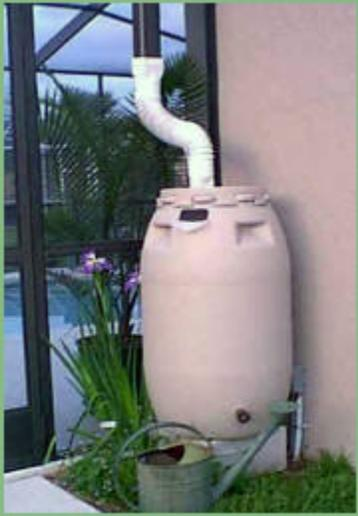
16. Place barrel on level, sturdy base. Direct downspout over the strainer. (Hooray, you now have a functioning rain barrel).
