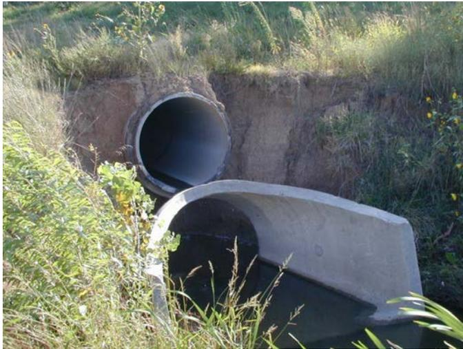
Photo 1. Storm Drain Conduits Need Restrained Joints
