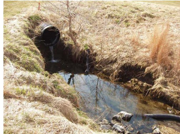
Photo 2. Outlets require erosion protection
