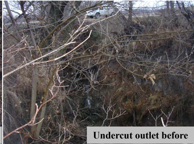
Undercut outlet before
