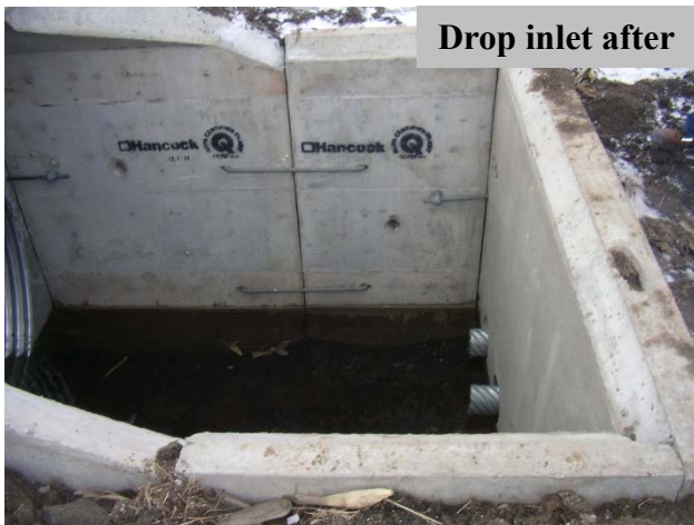
Looking upstream of drop inlet at filled gully after
