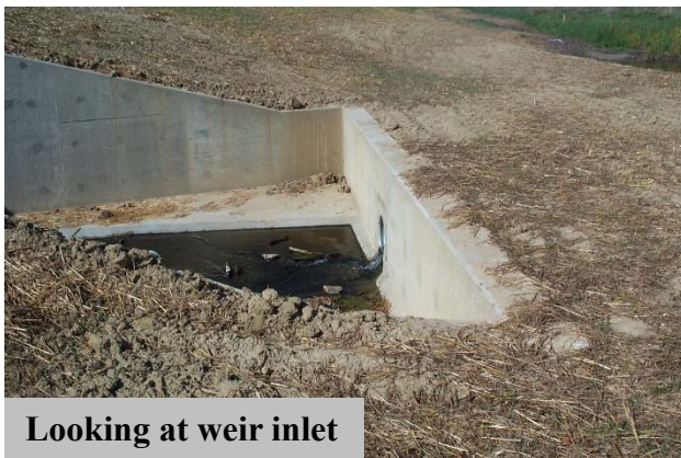
Looking through slope-tapered inlet
