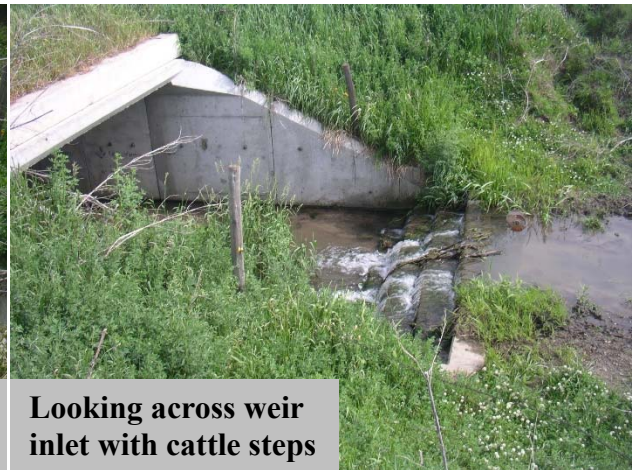
Looking upstream at weir inlet with cattle steps
