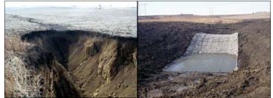
Left: A typical gully in western Iowa. Right: To replace an erosive gully, a gabion basket chute was built with cost share from the HCA's landowners structure program
