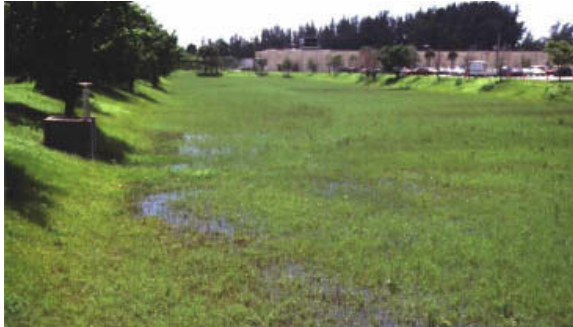
Source USGS File Photo Dry-detention
