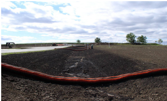
Open Channel with grade checks
